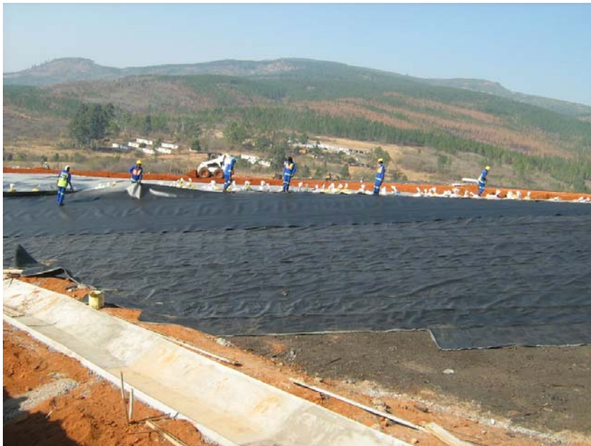
Installation of Geomembrane
