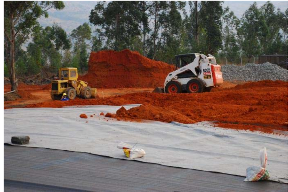
Placing of Cover Soil
