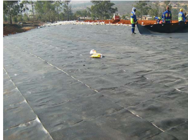
Installation of Laminated Hi-drain
