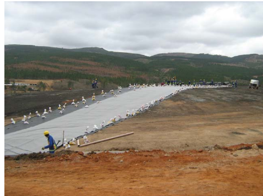
Installation of Geotextile
