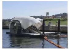
Plastic and other floating waste clog up waterways especially those that lead into the sea. This water wheel can either be powered by water currents or photovoltaic energy to drive a moving ladder system that lifts debris off the surface and into a holding barge which will take it be processed. Designed by waste engineers in Baltimore, it's applicable in harbours, dams, rivers wherever floating objects can be drawn into its uptake ladder. See more at: https://www.youtube.com/watch?v=RkQbcrzyAeE
