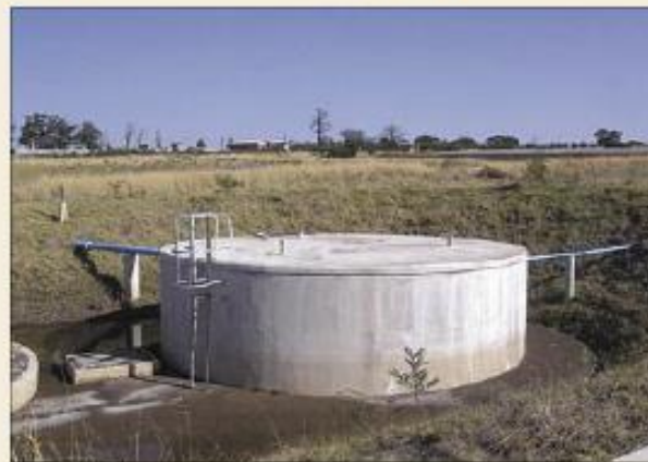
Construction of 700 klt leachate tank to collect leachate generated by the waste cell
