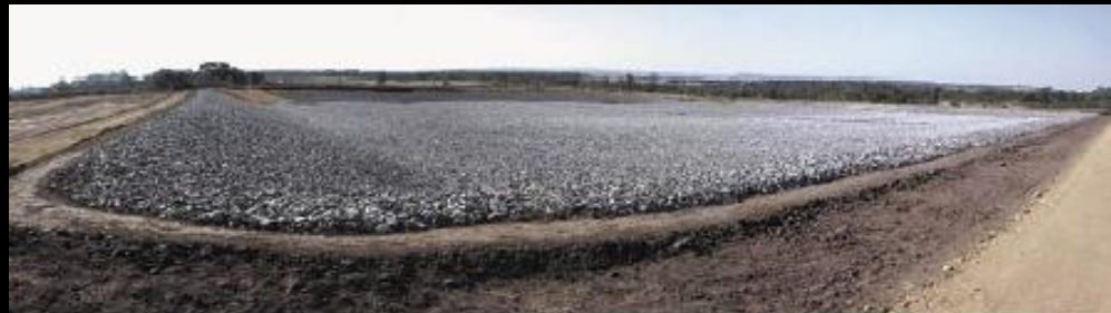
Completed construction of the first 2.5 ha capacity waste cell
