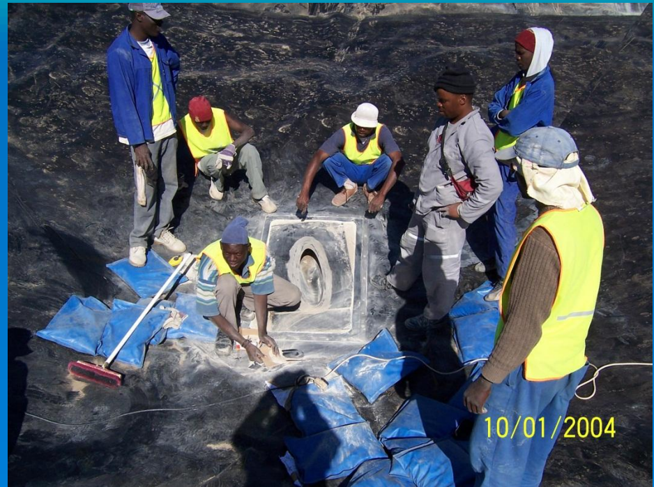
Battening of primary HDPE geomembrane to concrete pipe penetration base
