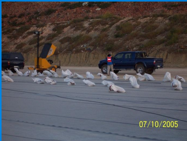
Preparing for early morning placement of sand protection layer
