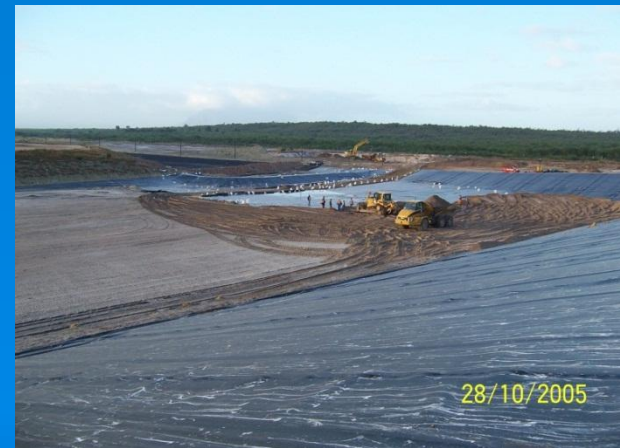
Note the smooth HDPE without wrinkles
