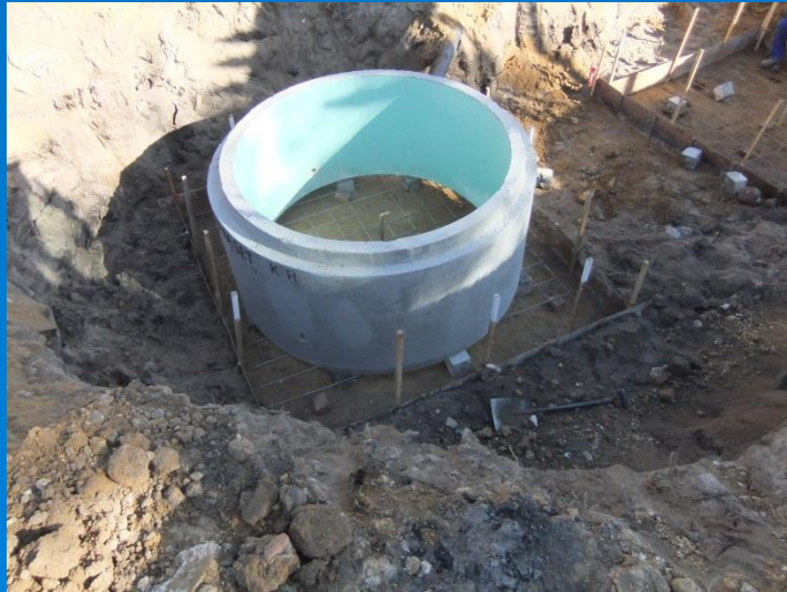
Concrete manhole ring with HDPE Anchor Knob sheet cast in
